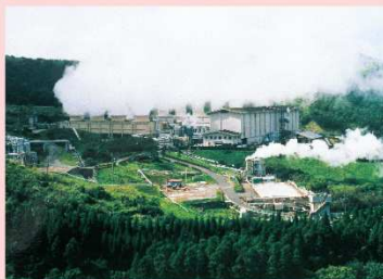
Geothermal Power Plants
